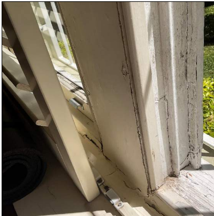
Photos 3 and 4 Represents: Deterioration of Timber Windows Within Unit 2
