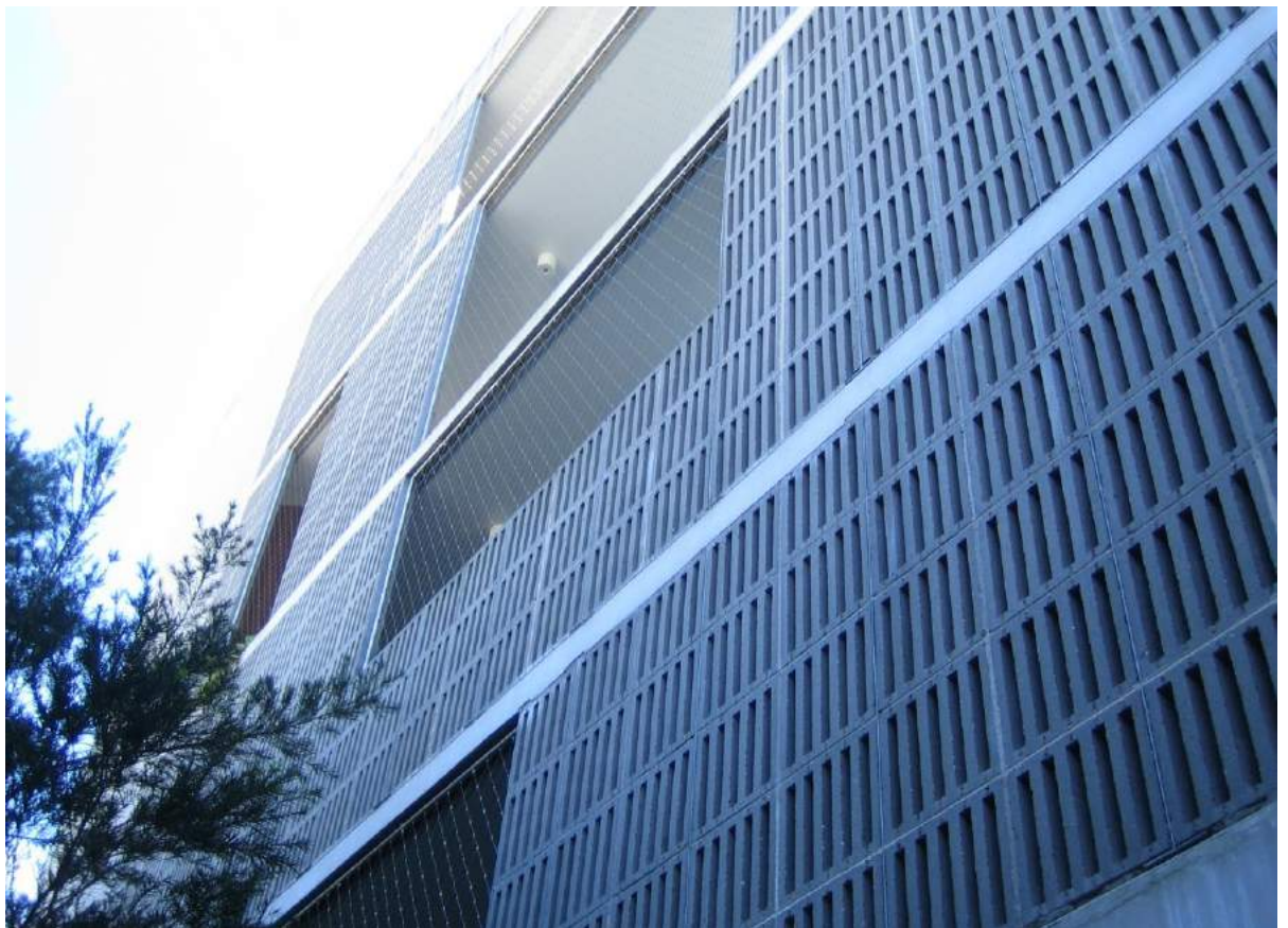
Photo No. 76: Upper levels of the western end of the southern elevation of Building B.
