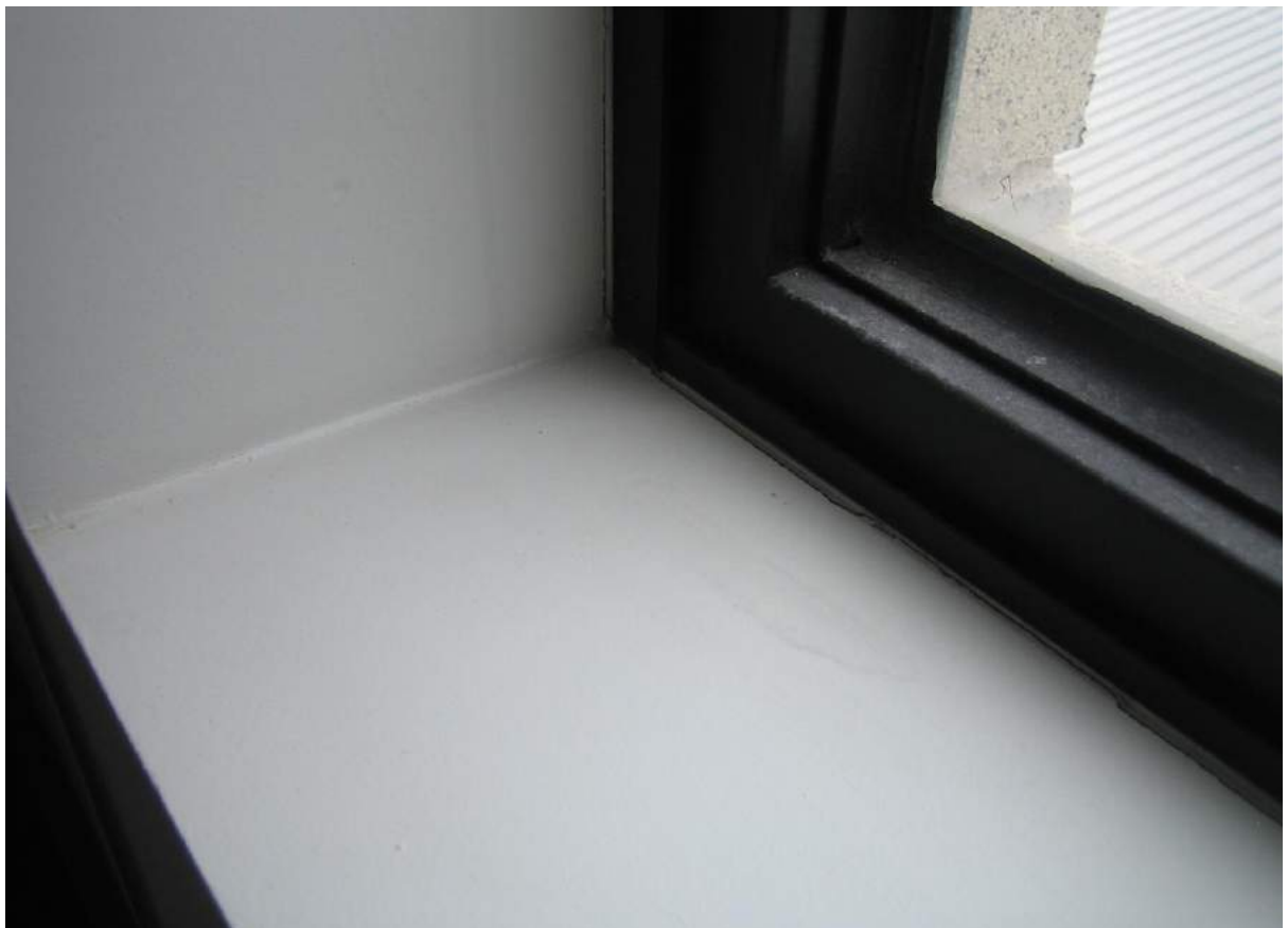
Photo No. 18: Water penetration and damage to the window sill in bedroom 1 in Unit 301.
