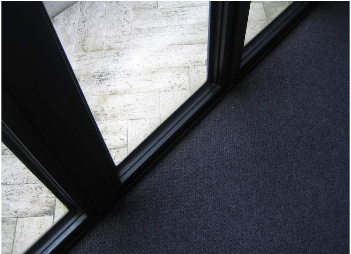
Photo No. 47: Water penetration and damage within bedroom 2 from balcony door in Unit 407.
