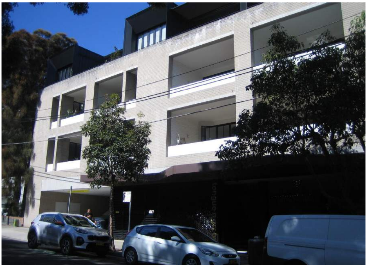
Photo No. 60: Eastern end of the northern elevation of Building A.
