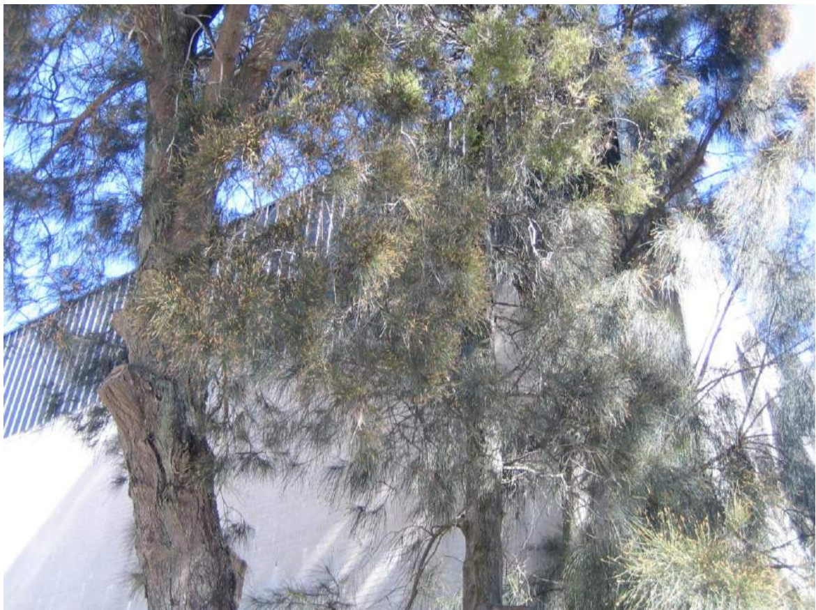
Photo No. 64: Northern end of the eastern elevation of Building A.
