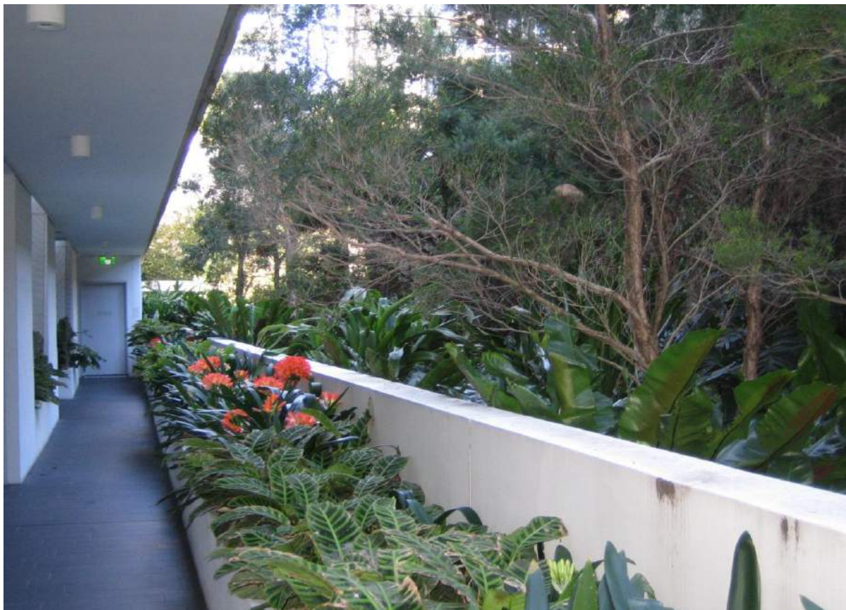
Photo No. 80: Lower levels of the ground level walkway in the southern elevation of Building B.
