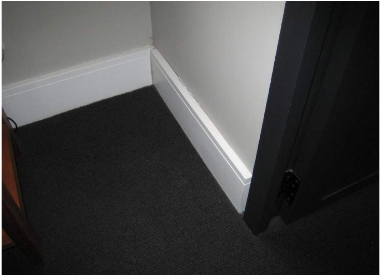
Photo No. 19: Water damage on the southern return wall in bedroom 1 in Unit 301.
