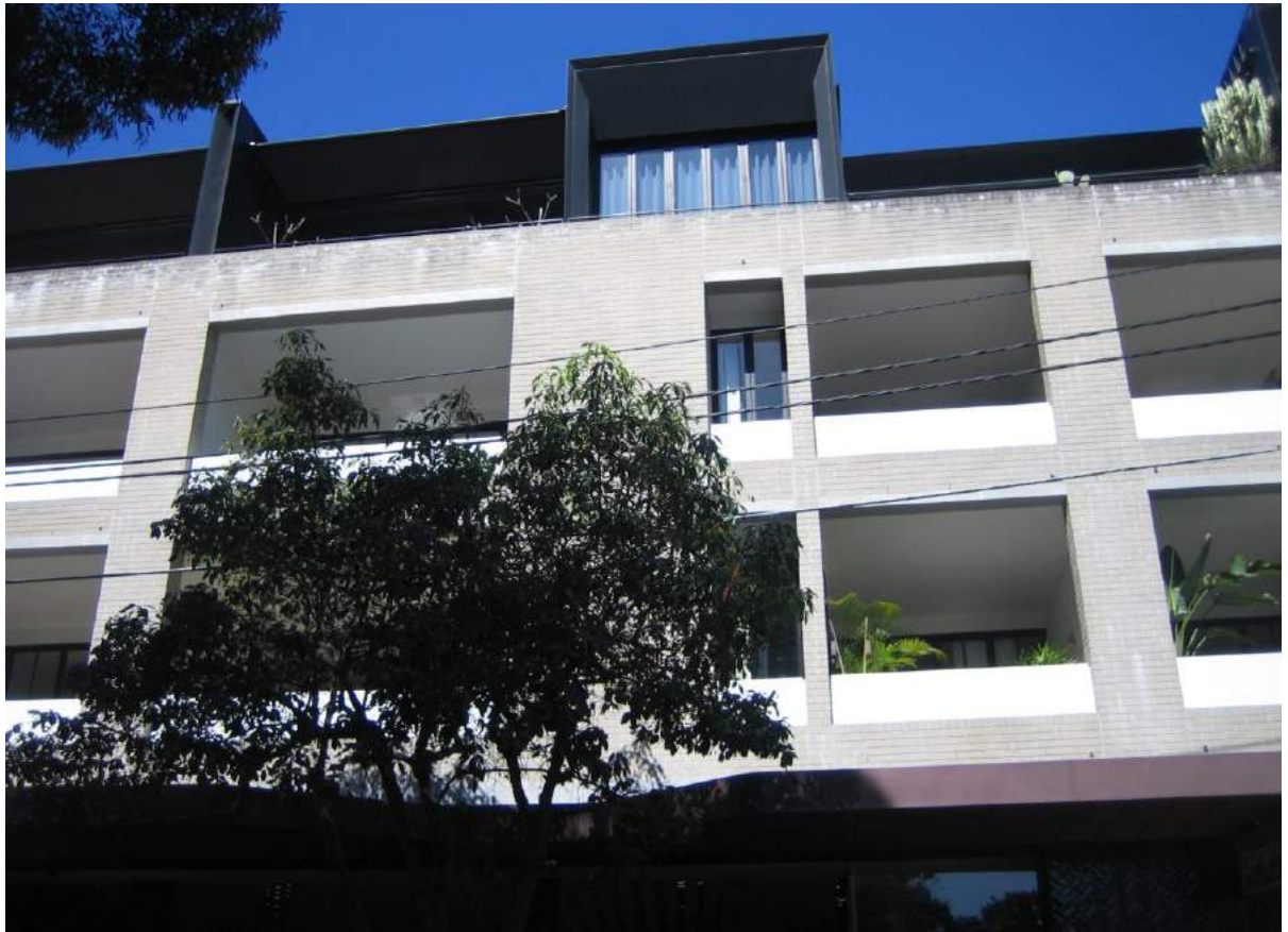
Photo No. 61: Middle section of the northern elevation of Building A.
