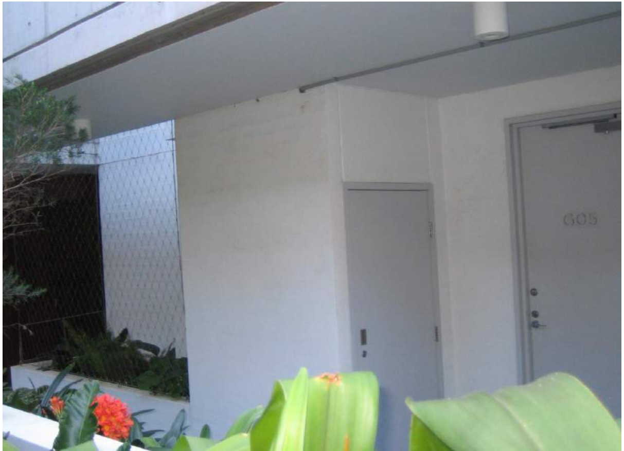
Photo No. 79: Lower levels of the western end of the southern elevation of Building B.
