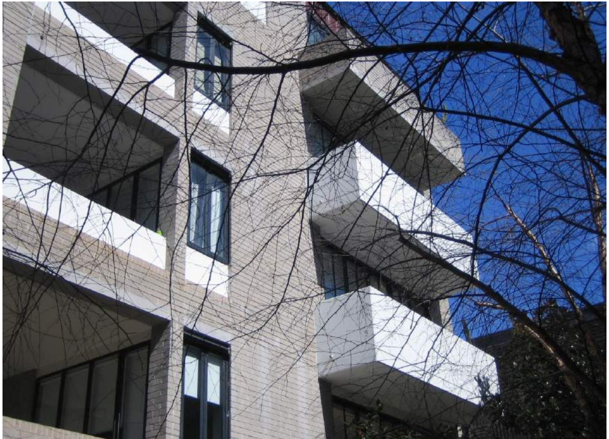
Photo No. 75: Western end of the northern elevation of Building B.
