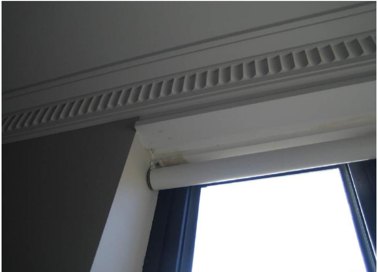
Photo No. 9: Water penetration in head of the eastern window in bedroom 1 to Unit 101.
