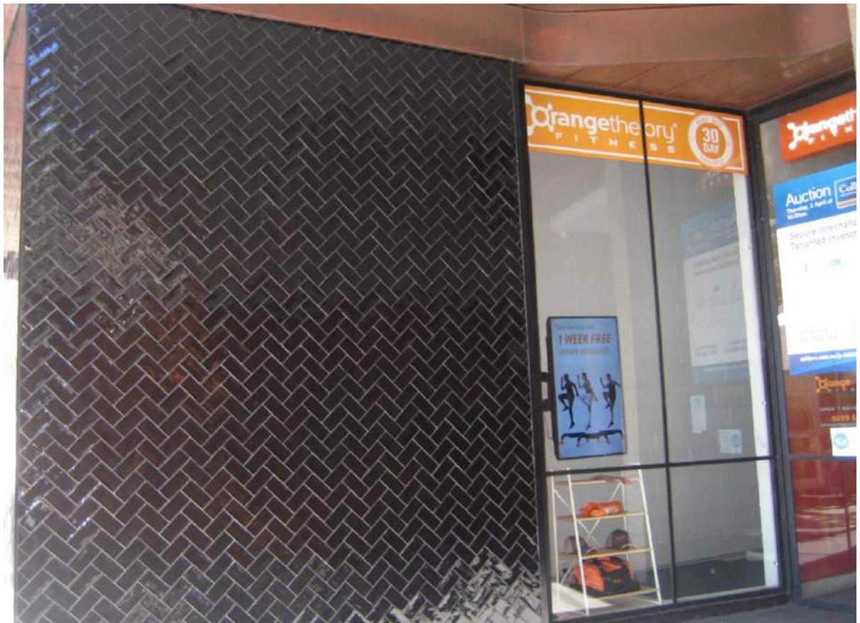
Photo No. 59: Main entry area in the western elevation in Building A.
