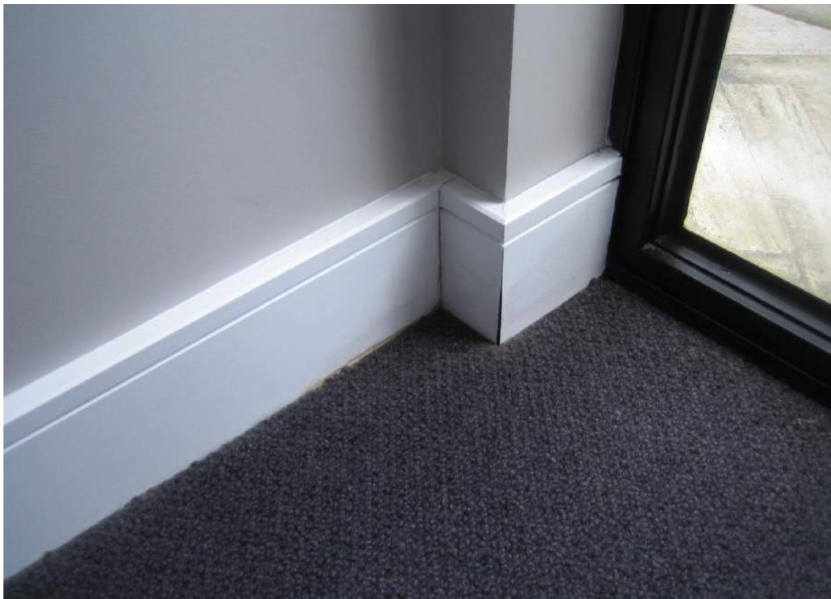
Photo No. 48: Water penetration and damage within bedroom 2 from balcony door in Unit 407.
