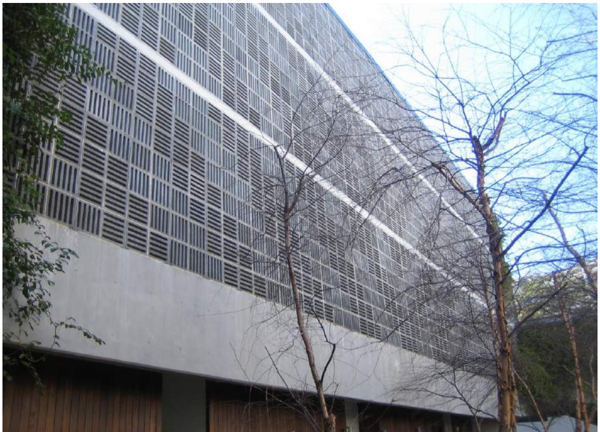
Photo No. 56: Eastern end of the southern elevation in Building A.
