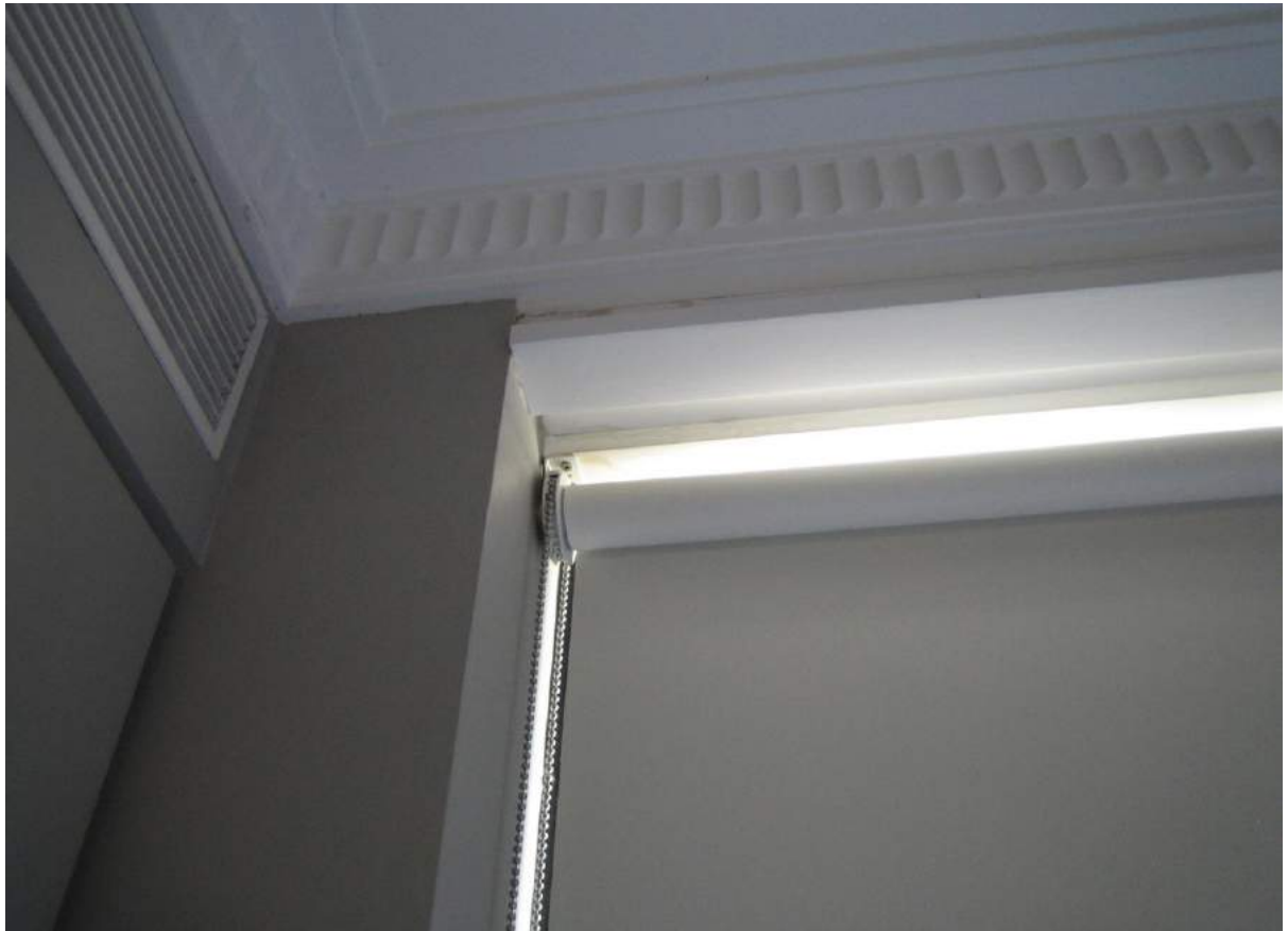
Photo No. 11: Water penetration in head of the eastern window in bedroom 2 to Unit 101.
