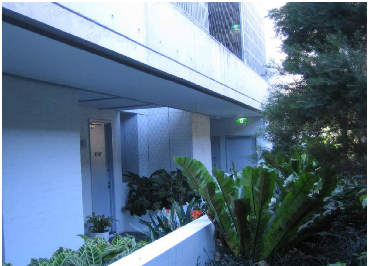
Photo No. 78: Lower levels of the eastern end of the southern elevation of Building B.
