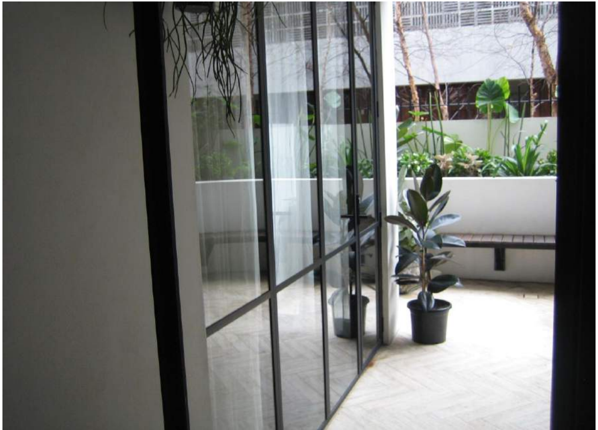
Photo No. 7: Glass wall/door configuration adjacent to N/E corner of bedroom 1 in Unit G05.
