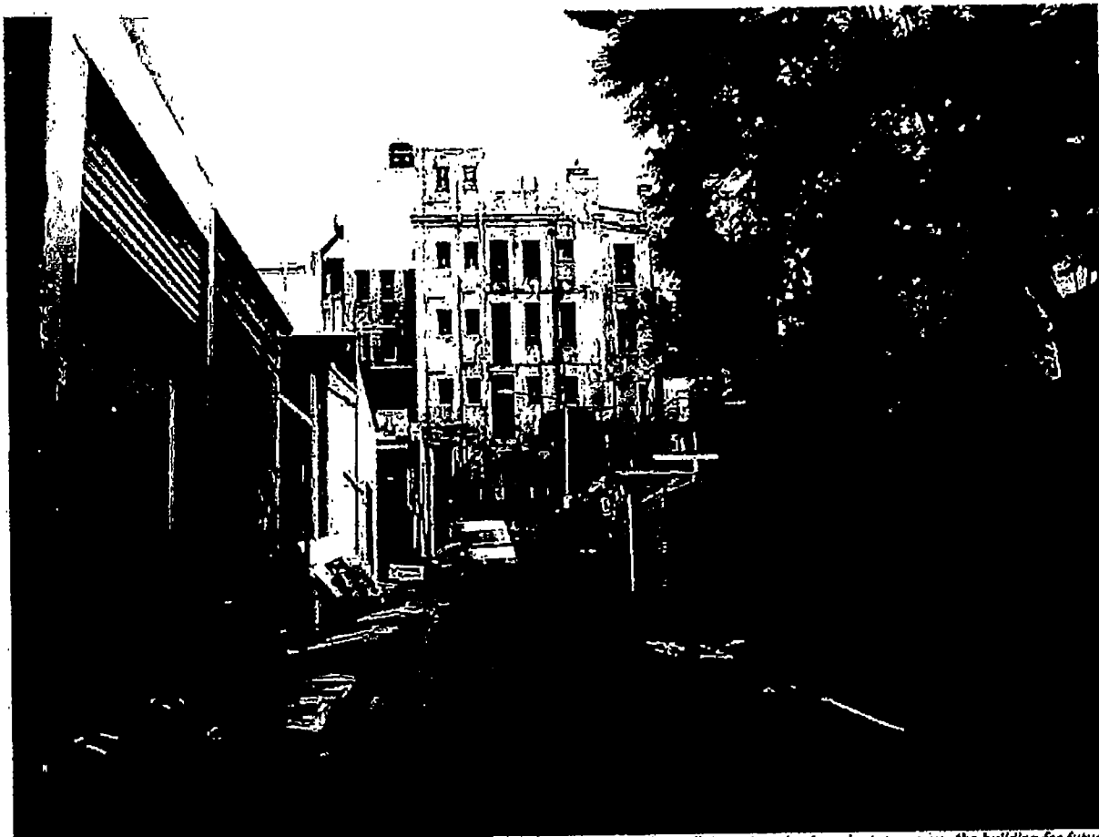
Figure 16: The rear elevation of Hotel Mansions presents an image of a building requiring immediate restoration in order to conserve the building for future generations.
